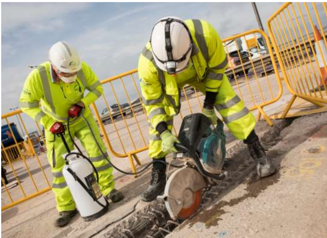
Preparing reinforced concrete 'deck end' joints for repair
