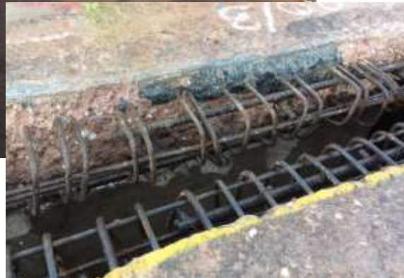
Concrete joint ready for repair after hydro-demolition
